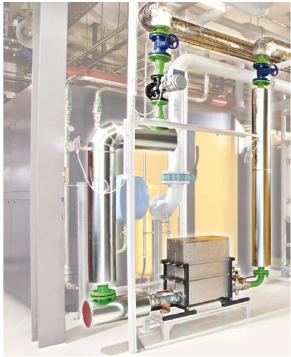
Figure 3. When dealing with existing systems, many compressors can be retrofitted with external heat exchangers for heat recovery.
