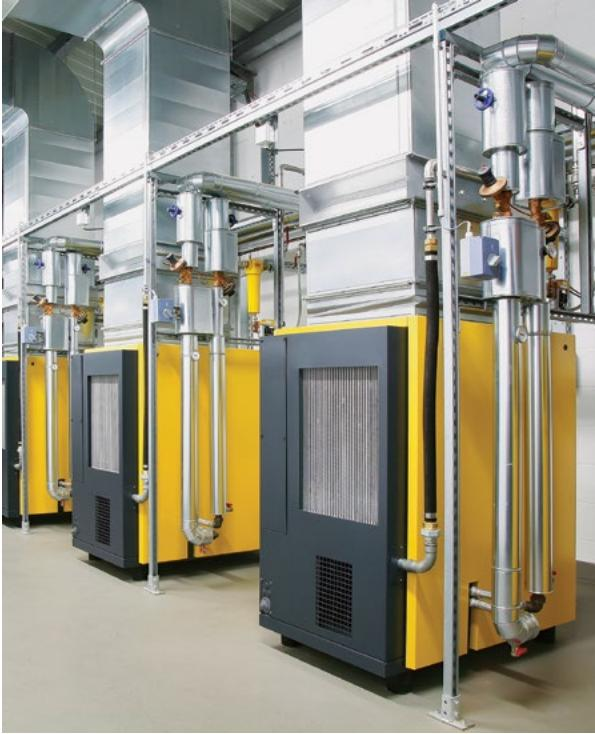
Figure 2. Ducting and tapping into the fluid circuit of compressors is an excellent way to utilize a compressor as a heat source and reduce operating costs.
