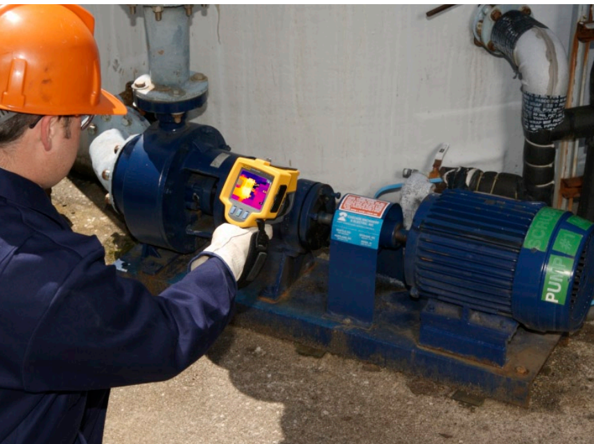
Take a baseline image of all motors, to compare over time, and then routinely look for abnormal hot spots on the motor, under full load.
