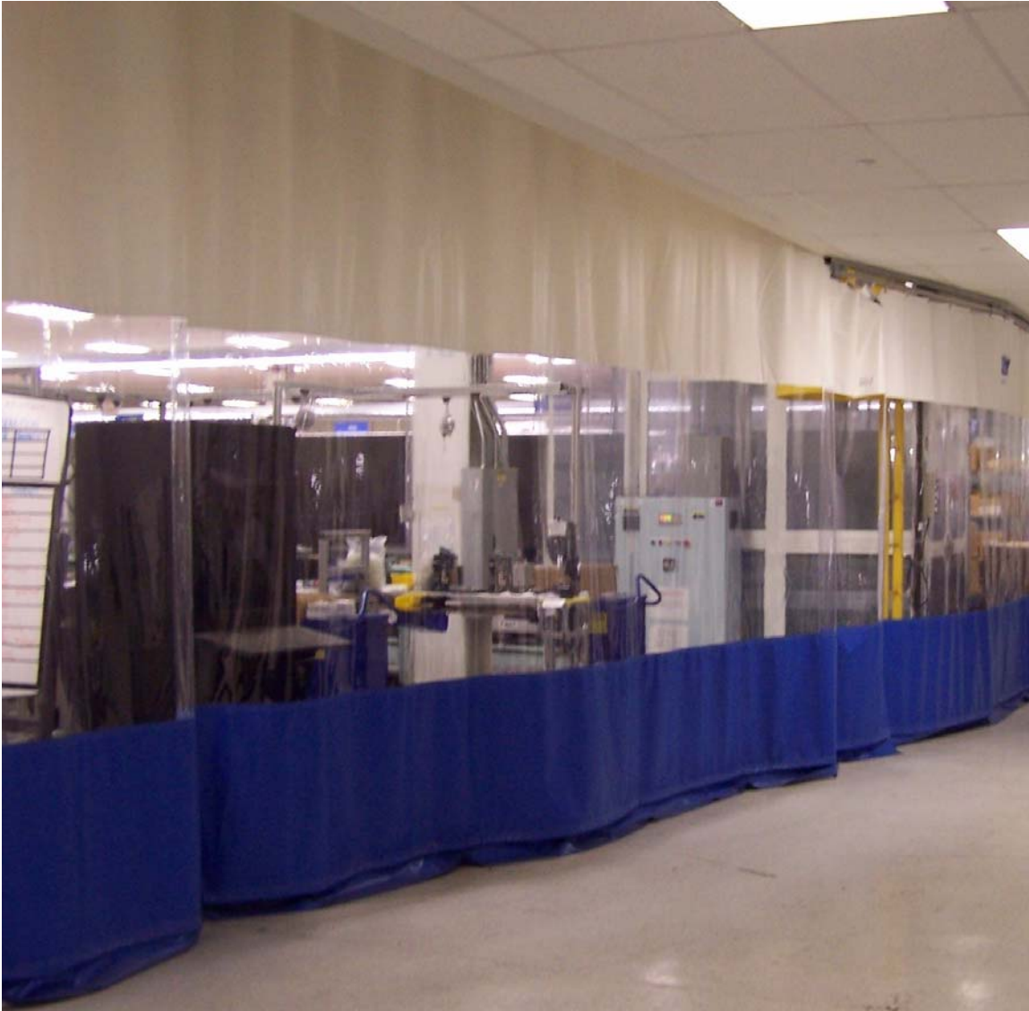
This 80'x120' area is enclosed by Goff's Curtain Walls to match the conditions of a class 10,000 cleanroom.
